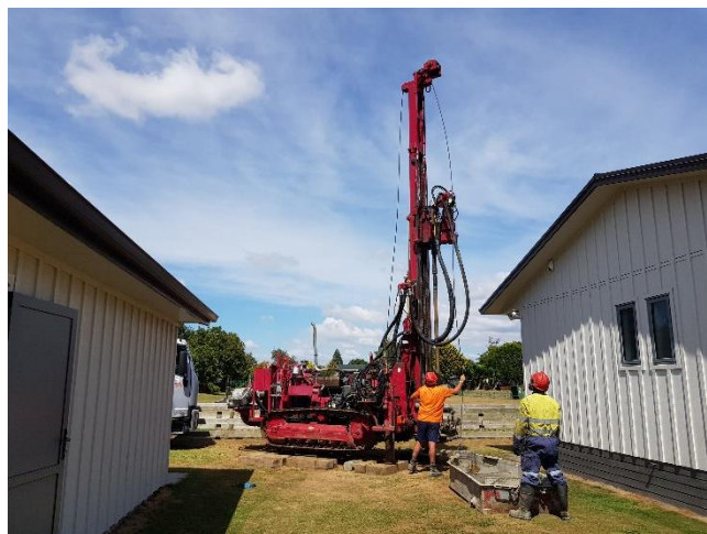
Drilling Rig in Position!
